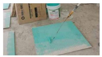
2 Apply a layer of **BEBOND BB1** on rear side of tile. Leave it to dry for about 30 mins
