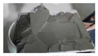
Apply ready mixed grout ( BEBOND BBBONDER + cement + water ) to the tile treated with BEBOND BB1
