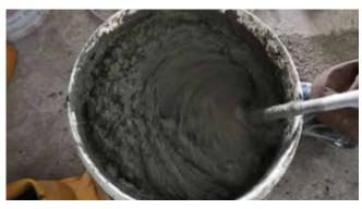
Pour 25kg cement into water and stir evenly (Additional mixing of up to 40% of fine sand is allowed).
