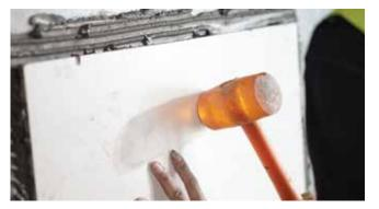
birect tilling on substrate treated with **BEBOND**BBPRIME.
